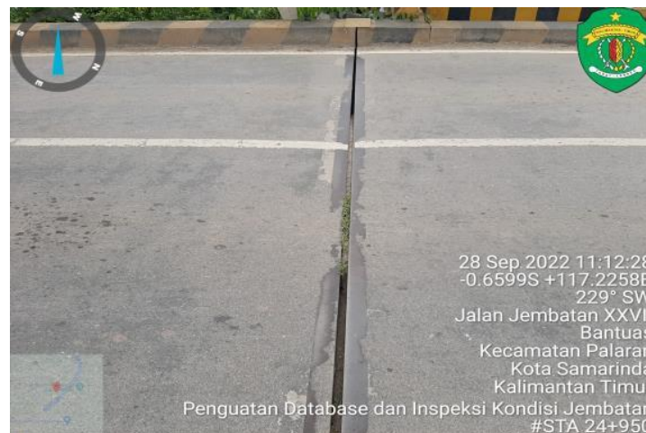
Gambar 5. Expansion join tabut menter isi pasir
